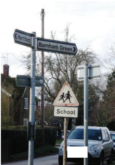
Figure 24: Collection of road signage, could the necessary signs be accommodated on less poles?
