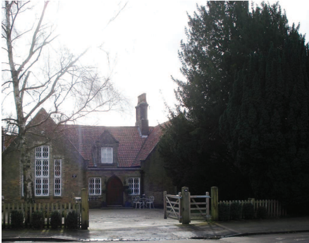
Figure 22: Trees to the front garden of 10 Lower Green
